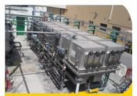
**DGF/DNF** - Dissolved Gas flotation unit using nitrogen-gas or biogas in the aeration system
